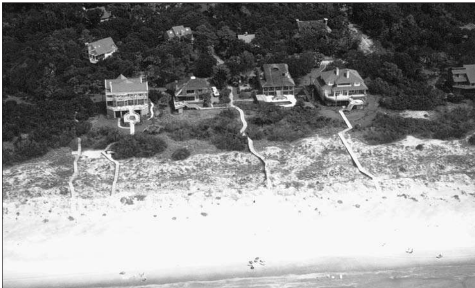
Figure 3-8. Coastal development well-suited to the land: generous setbacks, in combination with deep lots and avoidance of dune areas, should afford protection from erosion and flooding for years to come.
