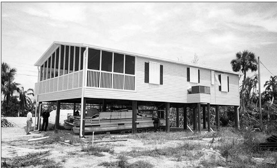
Figure 8-4. Manufactured home on a pile foundation.
