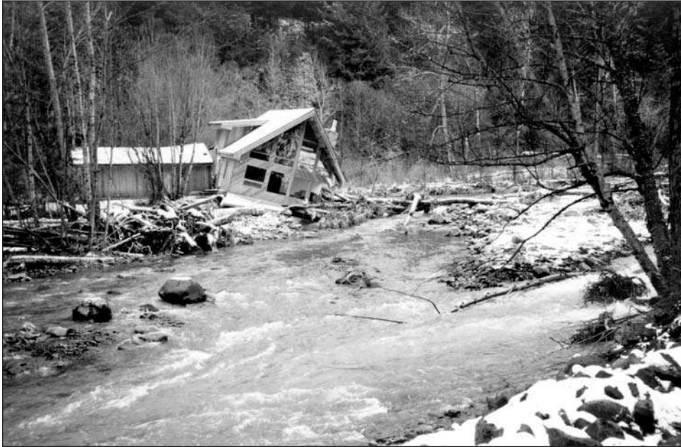
Figure C-7. Home damaged along a stream subject to flash flooding due to surrounding mountainous terrain.
