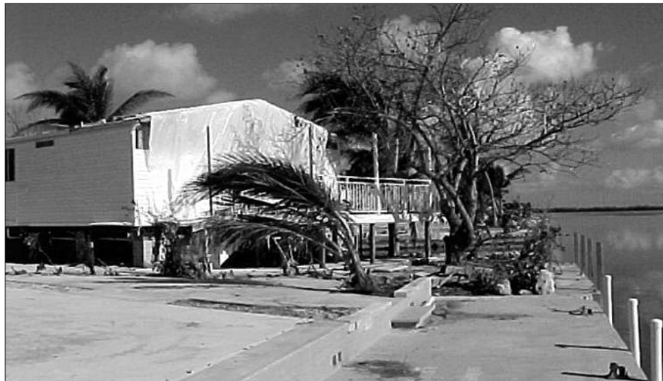
Figure 1-5. Manufactured home in Cudjoe Key, Florida, built and installed after 1994, survived Hurricane Georges with only minor damage caused by the loss of an awning. The older manufactured home on the lot next door was destroyed by high winds and coastal surge.
