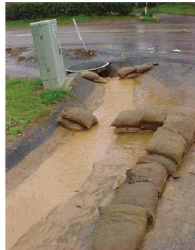
Figure 5. Make sure storm drain inlets are protected.
